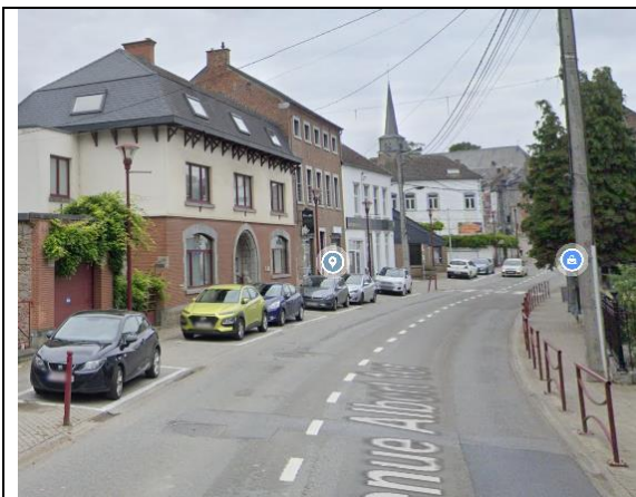
Figure 140 : Avenue Albert 1, Gerpennes (Source : Google Maps)
